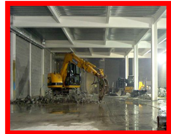
Zara Escalator installation
