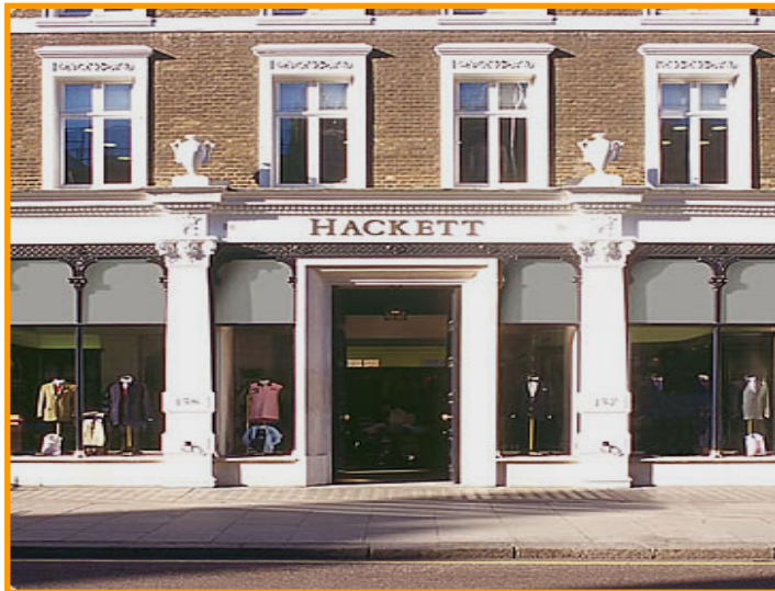
Project: Hackett Integration & Implementation: Shopspec uk,, Our Performance: Cost & Project Management
